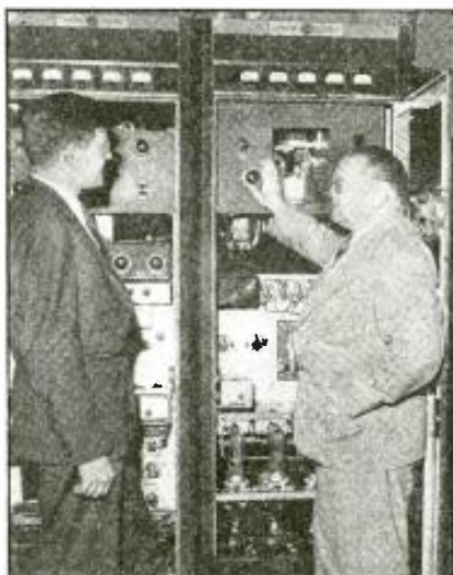
Assistant engineer D. E. Chambers and C. A. Priest, Engineer Radio Transmitter Dept. (l. to r.), inspect new G. E. 1 kw. F.M. transmitter on test floor at Schenectady. They point out how all parts are accessible for inspection, test or repair.
